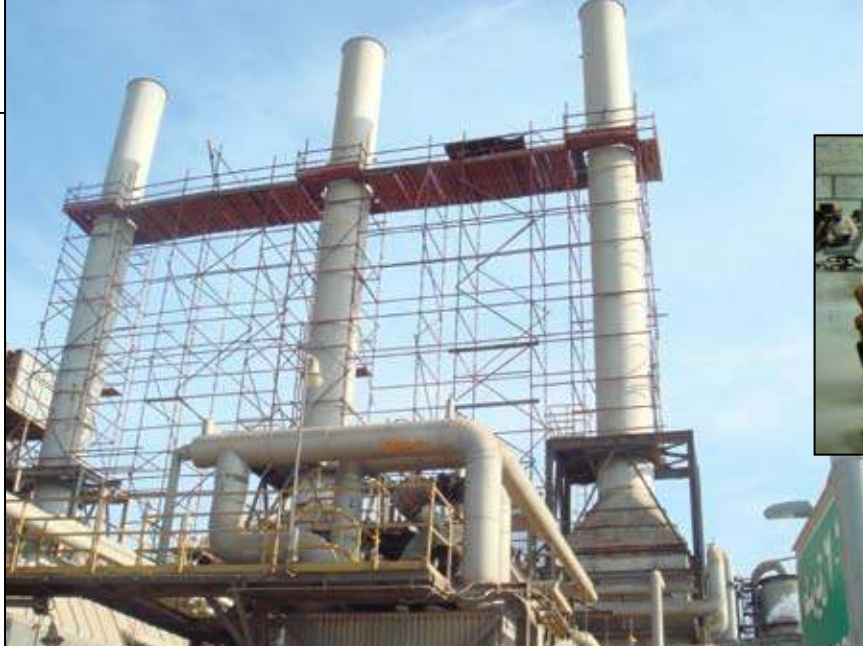
FIGURE 2. PEMS was implemented on the boiler stacks at Arrazi, three of which are shown here
