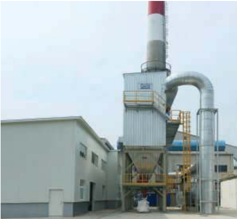
FIGURE 4. Shown here is a catalytic hot-gas filtration system installed in the glass industry by Dürr
